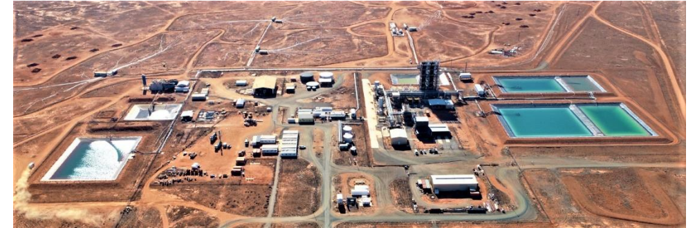
Honeymoon Processing Plant and Wellfields, South Australia
