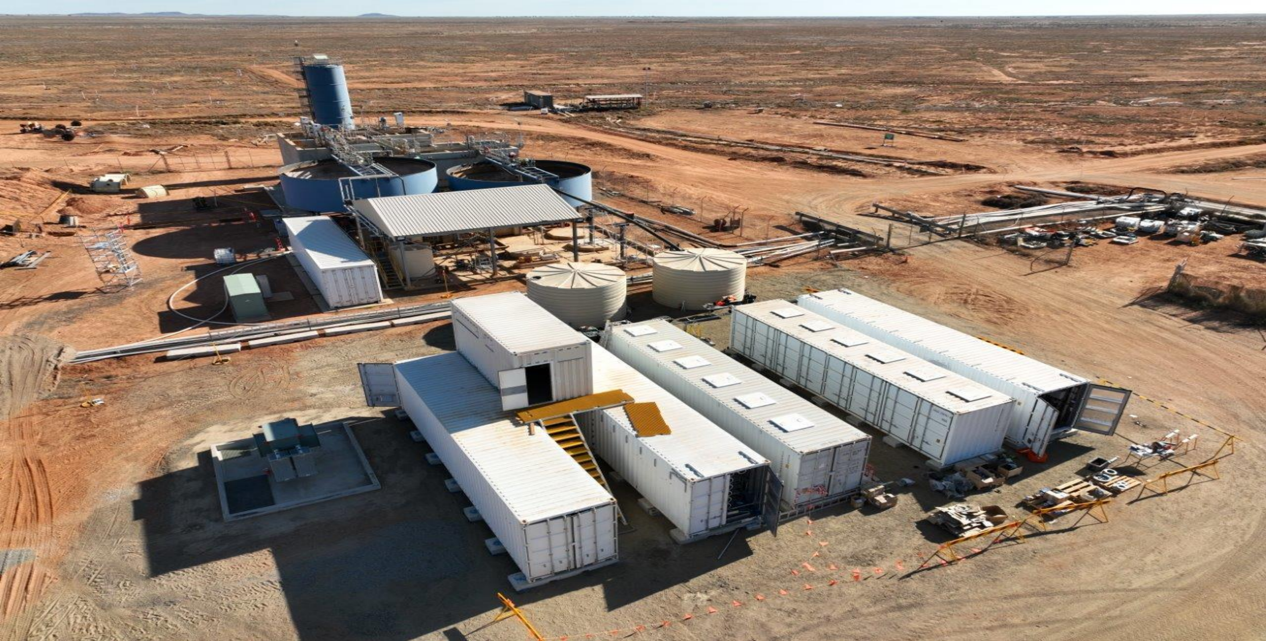
RO and Water Treatment Plant
