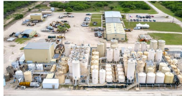
Alta Mesa Central Processing Plant, Texas, USA
