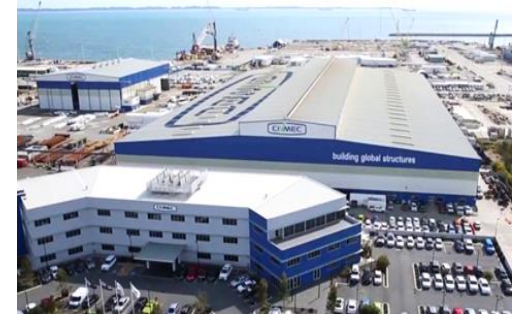
Steel fabrication and plant modularisation
