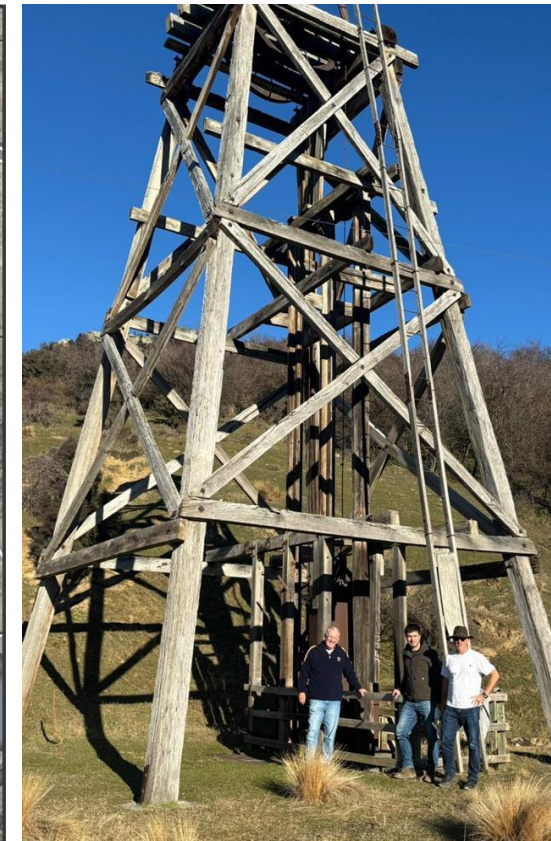
Headframe at Oturehua's Golden Progress Mine
