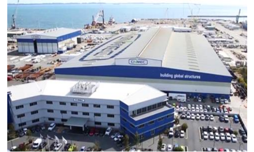
Steel fabrication and plant modularisation
